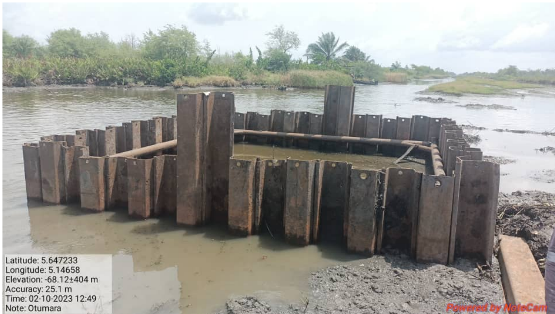
COFFERDAM CONSTRUCTION FOR JIV/IC REPAIR BY SPLIT TEE INSTALLATION AT OTUMARA
