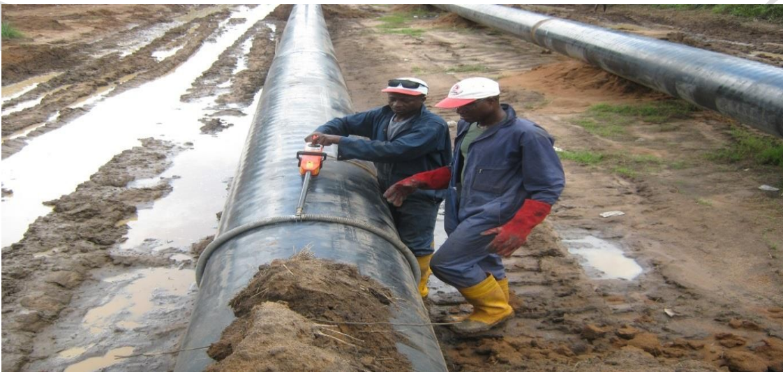
HOLIDAY DETECTION TEST ON WRAPPED PIPE JOINT
