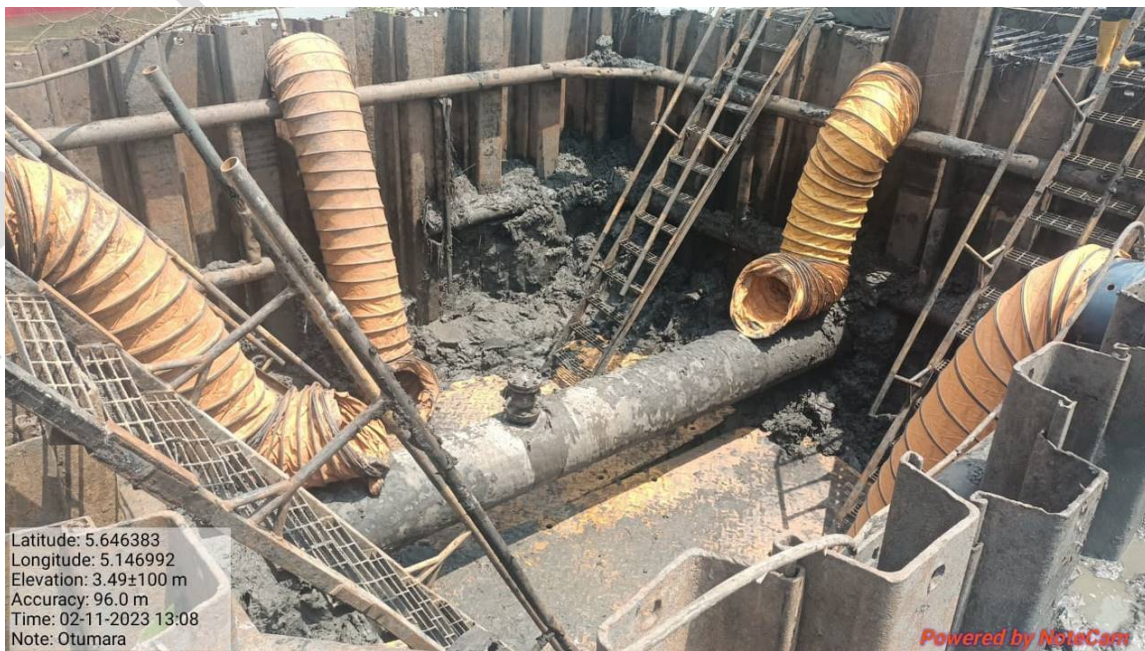
COFFERDAM CONSTRUCTION FOR JIV/IC REPAIR BY SPLIT TEE INSTALLATION AT OTUMARA WITH ALL SAFETY MEASURES IN PLACE
