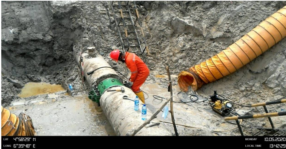
TORQUE ACTIVITY ONGOING ON 20" KCTL AT IHUOWO
