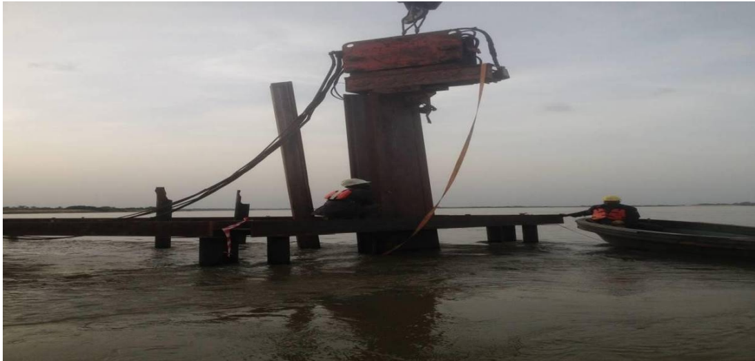
PILING WORKS USING VIBRO-HAMMER
