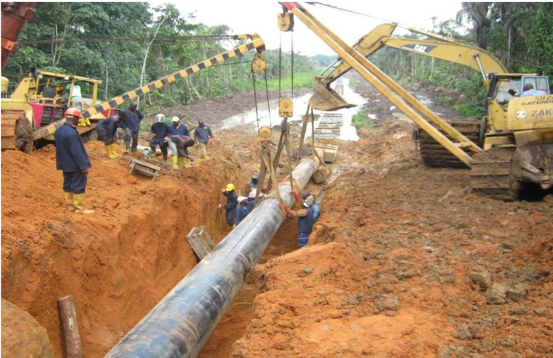
LOWERING OF 24" GAS LINE WITH THE HELP OF SIDE BOOMS AND EXCAVATORS
