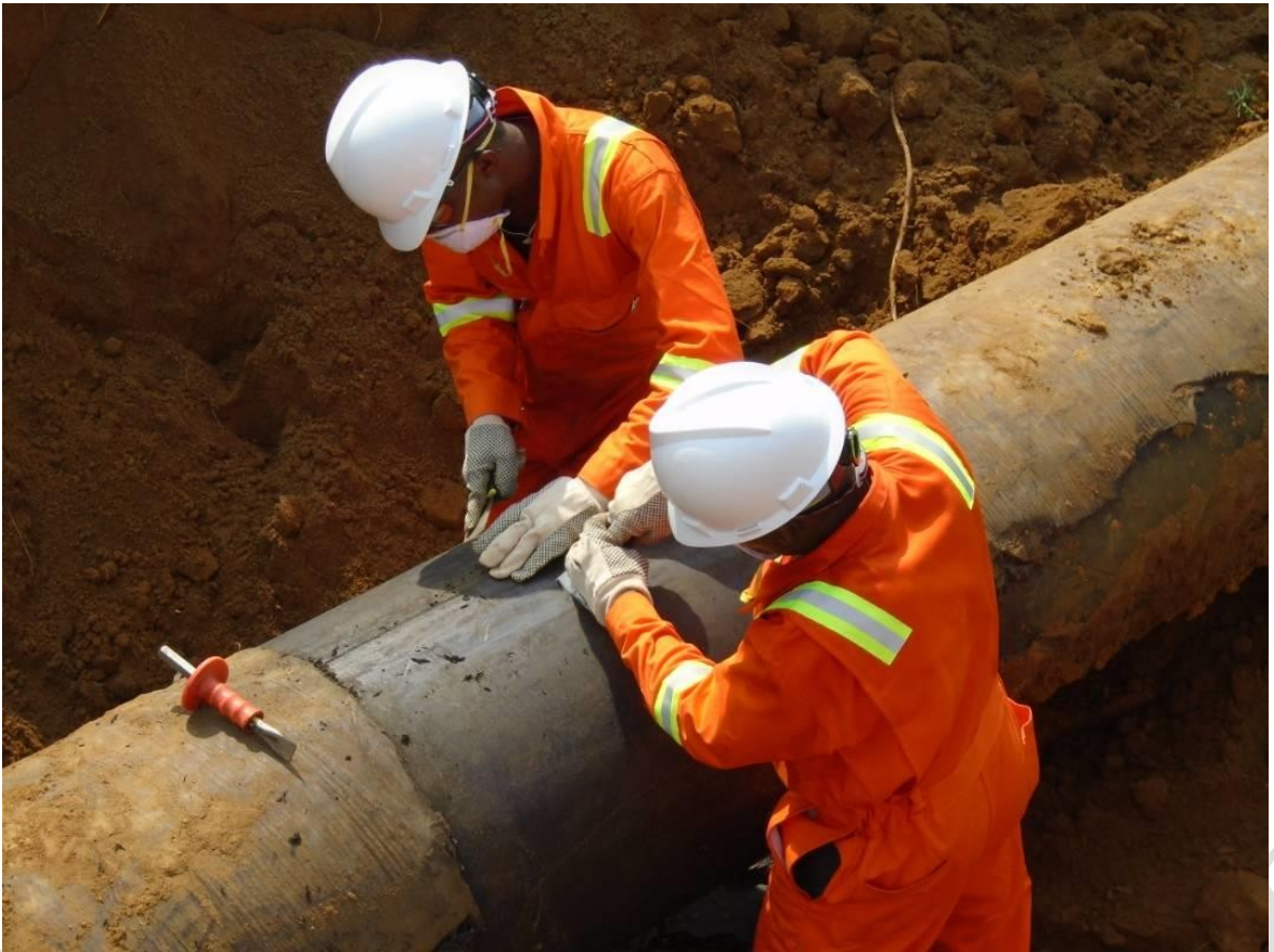
De-coating activity on TNP line
