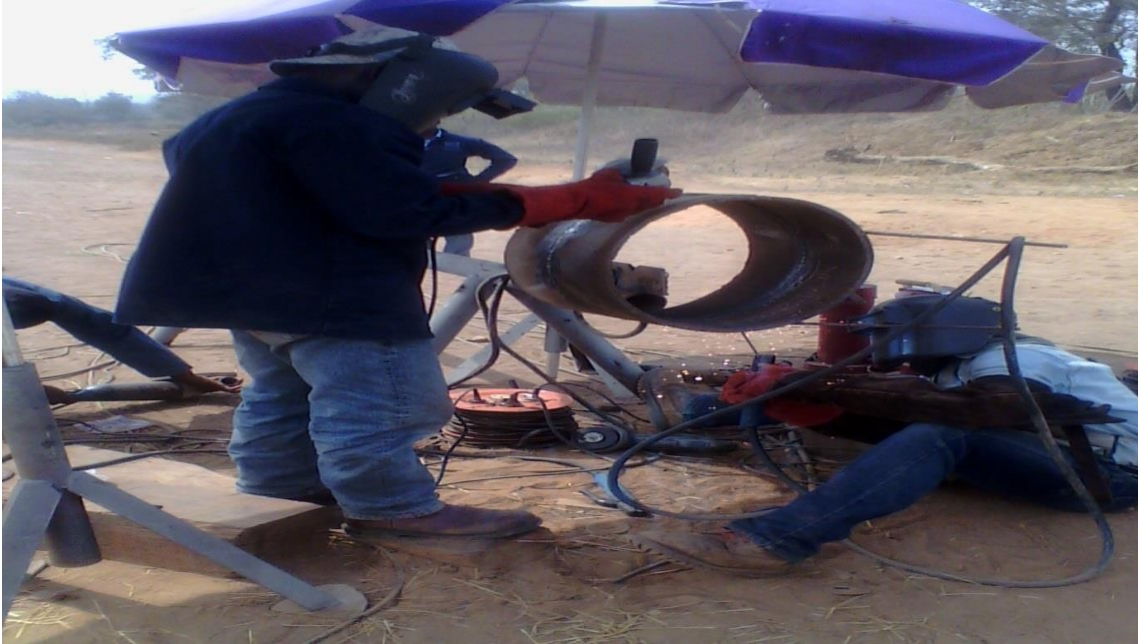
WELDERS UNDERGOING PROCEDURE TEST
