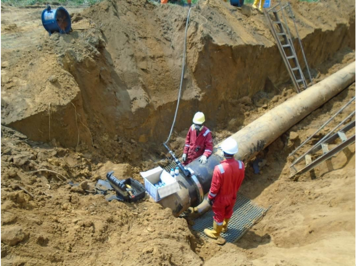
COLD CUTTING ACTIVITY ON TNP LINE AT BOTEM
