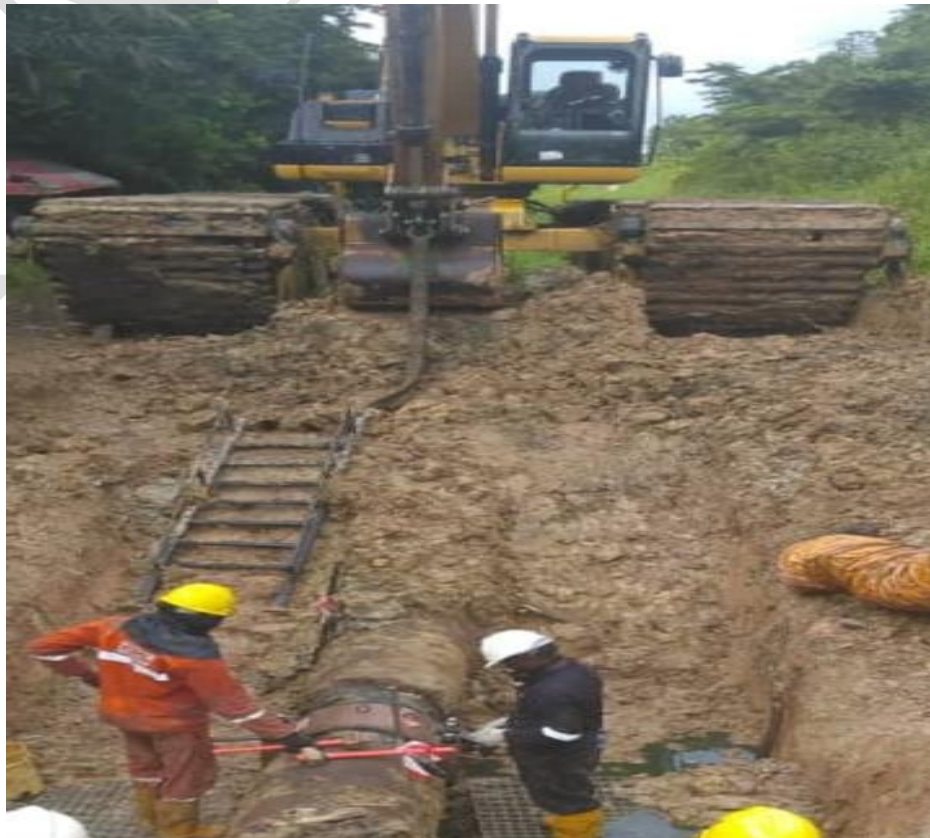
CLAMPING ACTIVITY ONGOING ON 20" KCTL AT AMINIGBOKO
